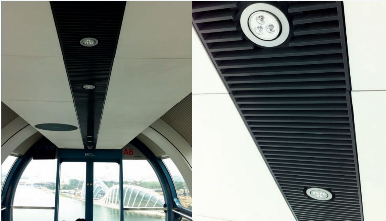
HO-LEDs are illuminating the world's largest ferris wheel in Singapore.
